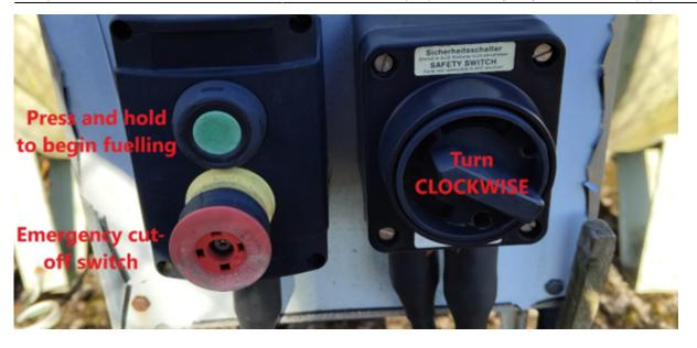
Unlock the gate and remove the padlock from the main isolator switch. Turn the isolator switch clockwise until it clicks.
