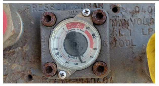
**Note:** The tank's gauge shows the pressure inside the tank. Around 60 is full.
